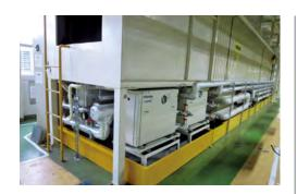
Introduction of heat pumps in the precoating process
